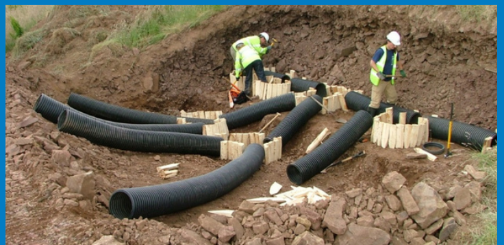
Above: installing custom built setts as habitat for local badgers
